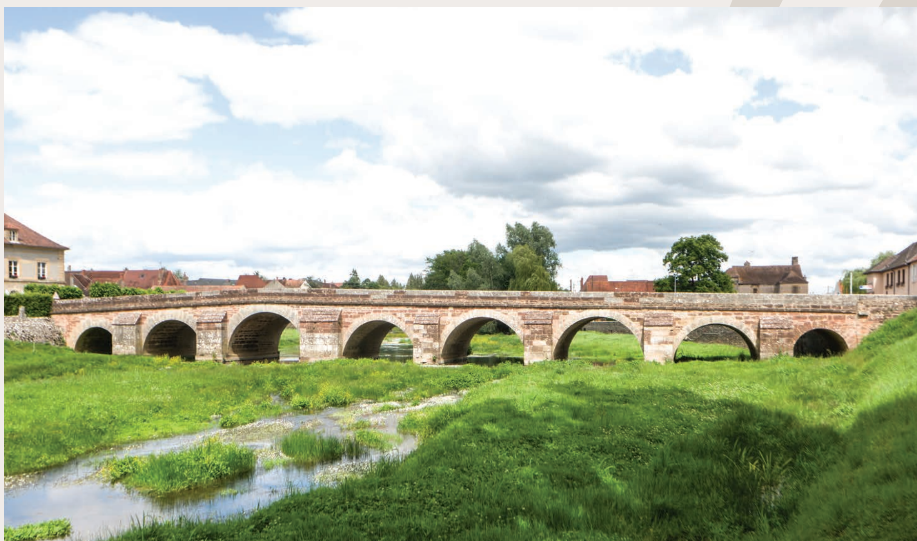
Pont aux 8 arches © G.Beurdeley
